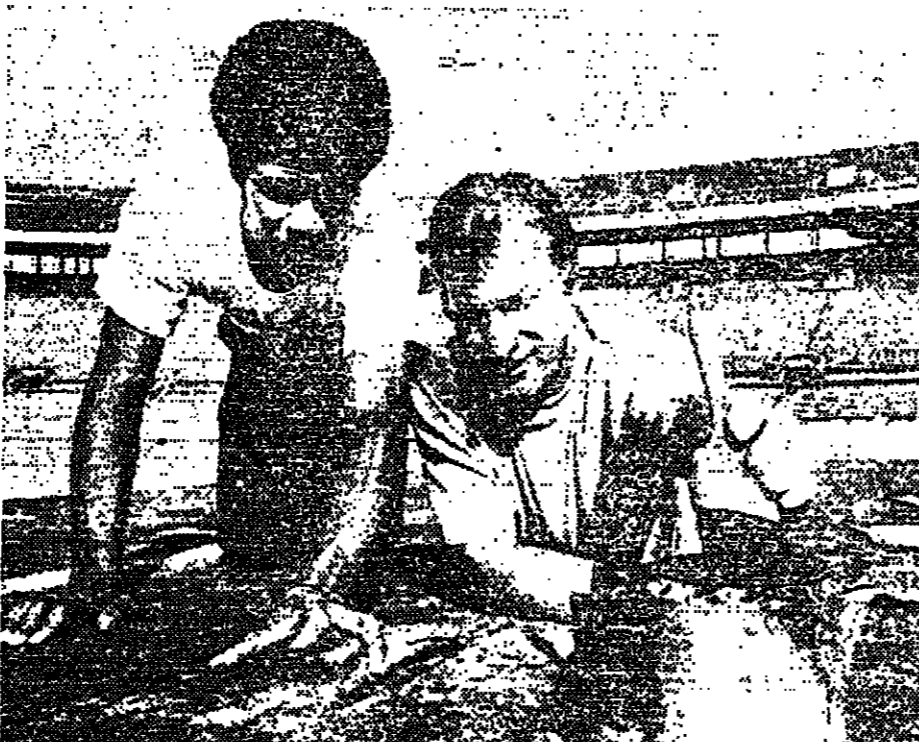
George Toma, the Kansas City Chiefs' groundskeeper, prepares to glue a loose seam of artificial turf of Orange Bowl, scene of tomorrow's Super Bowl game. Toma, who has made field ready for all previous Super Bowls, has vowed success for this game as well.
